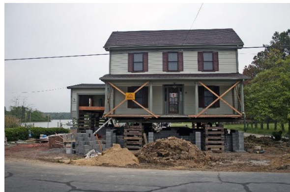
Photo 6.2 – Elevated Structure
