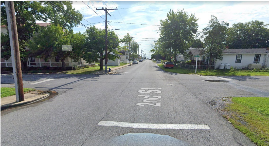
Photo 42 - Erie Avenue and 2nd Street
