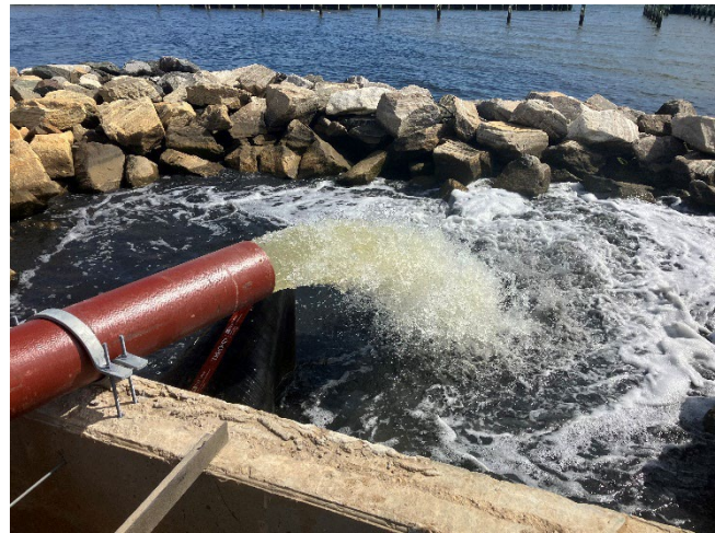
Photo 11 - New 5th Street Pump Station Outfall
