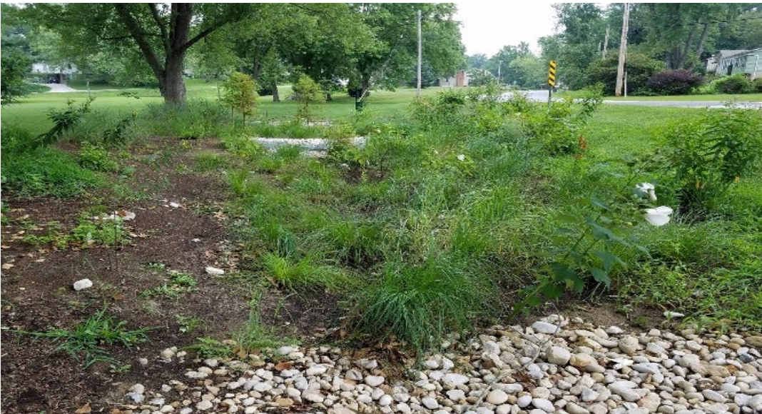
Photo 49 - Bioretention Facility
