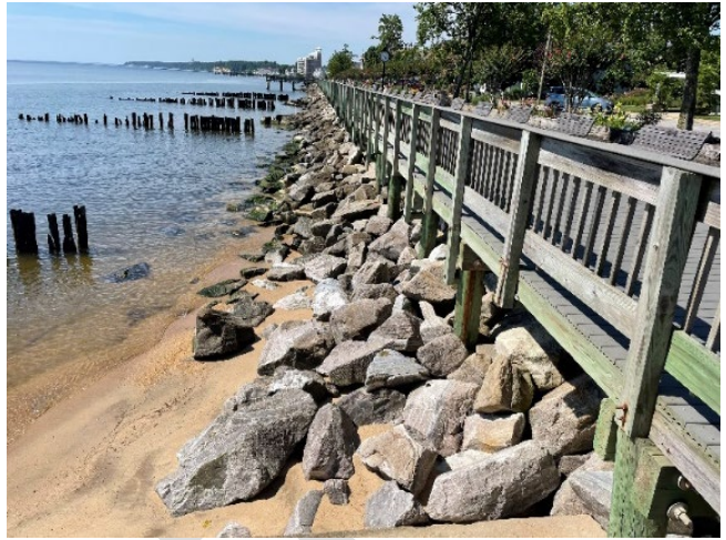
Photo 7 - Revetment along Boardwalk
