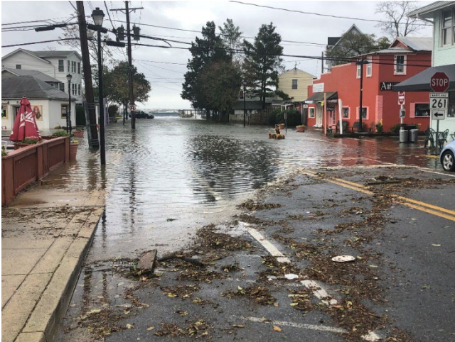
Photo 23 - 7th Street at Bay Avenue – Looking East
