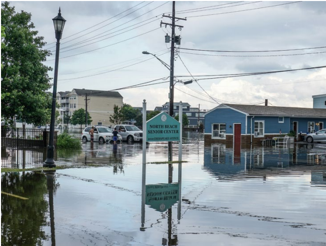
Photo 28 - Chesapeake Avenue at 3rd Street - Looking North
