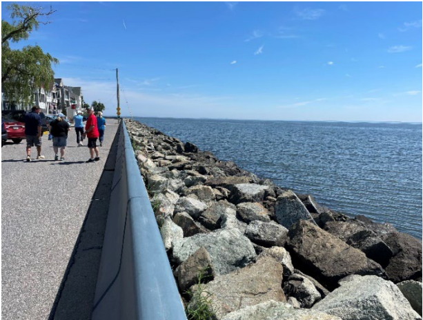
Photo 16 - Revetment and Jersey Barriers along Atlantic Avenue
