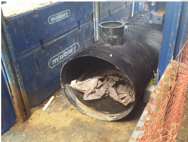
Photo 47 - Pipe Replacement
