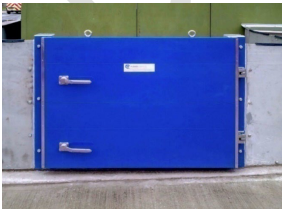
Photo 45 - Stop Log Gate along Concrete Wall
