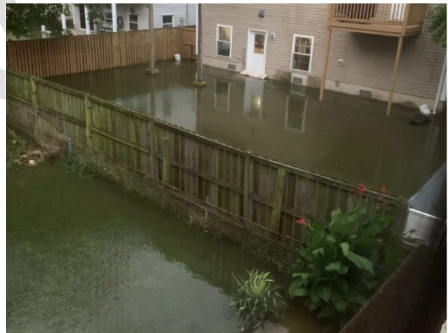
Photo 3 - Flooding from Storm Surge
