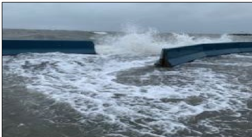
Photo 18 – Jersey Barrier moved during storm event
