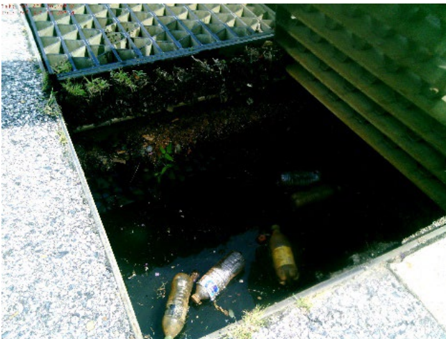
Photo 12 - Backwatered System with Trash
