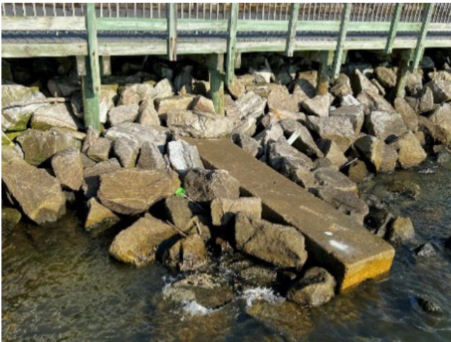
Photo 10 - Outfall Perpetually Backwatered
